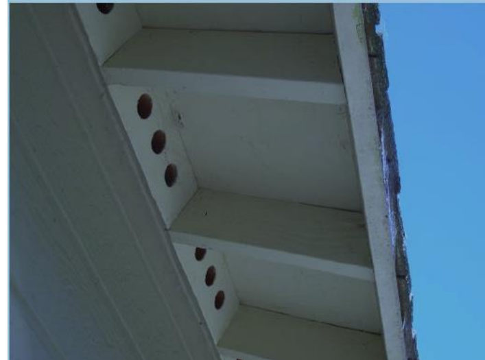
Unenclosed eaves Vents
