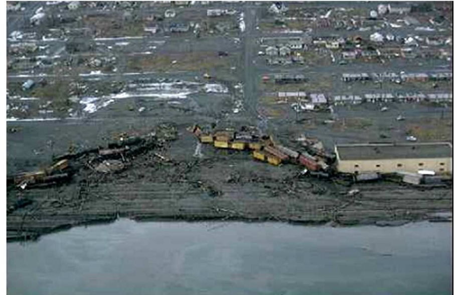
Tsunami damage along Seward's waterfront from 1964 M9.2 Alaska earthquake
