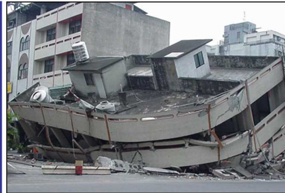
1995 M7.4 Kobe Earthquake, Japan
