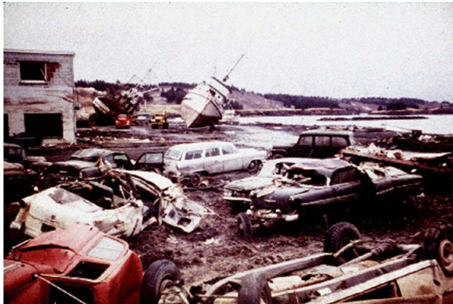
Tsunami damage along waterfront on Kodiak Island from 1964 M9.2 Alaska earthquake
